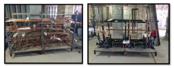
These racks allow workers to easily transport large amounts of preassembled piping systems from the trailers they are brought to site on and then rolled onto a material hoist or service elevator to bring them to the proper floor for installation. Once at their proper location the pieces are taken off the rack and lifted into place where the final connections are to be made.
